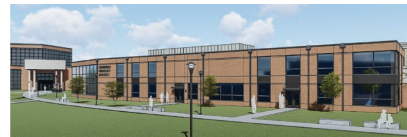
The new addition to Callan will house classrooms, labs, and faculty offices for our new Master of Athletic Training and PA* programs, as well as a new weight room and team room for our student-athletes.
