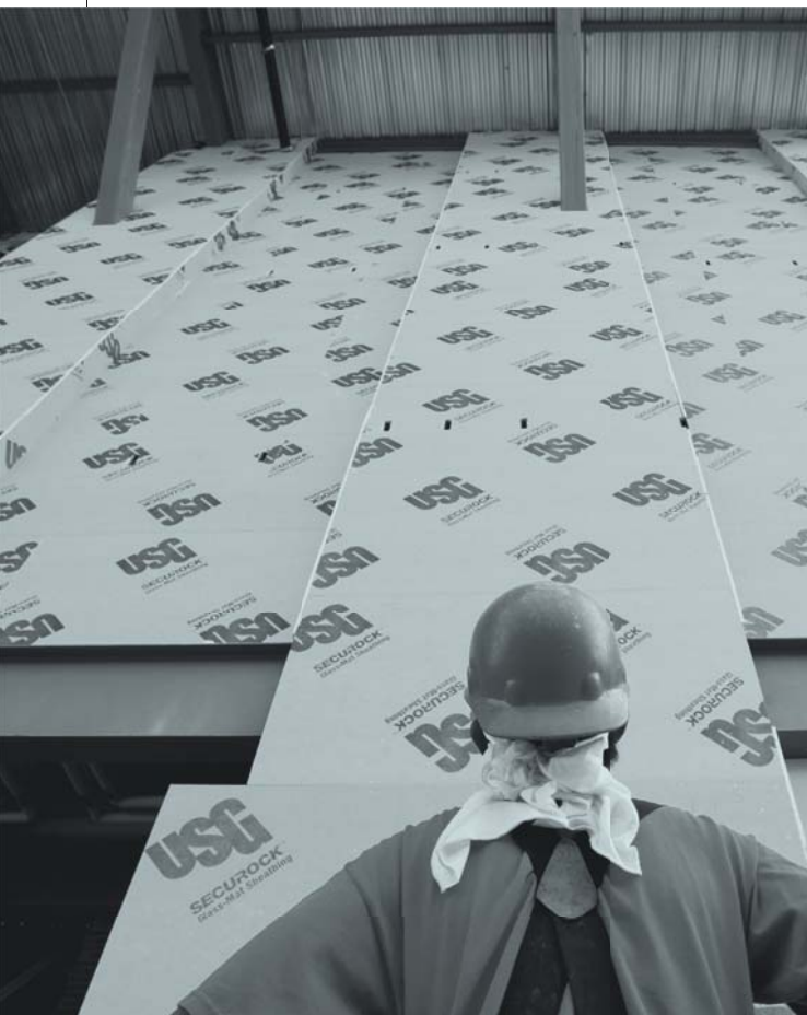
USG Securock Brand Glass-Mat Sheathing protects building exteriors during the construction process at a project at the University of Tennessee.
