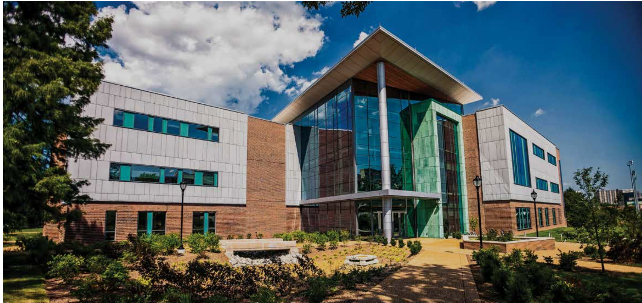
ABOVE: THE INTERDISCIPLINARY SCIENCE AND ENGINEERING BUILDING BELOW: A RENDERING OF THE JESUIT CENTER
